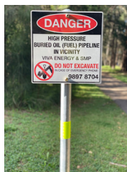
Pipeline easement marked by warning signs.
