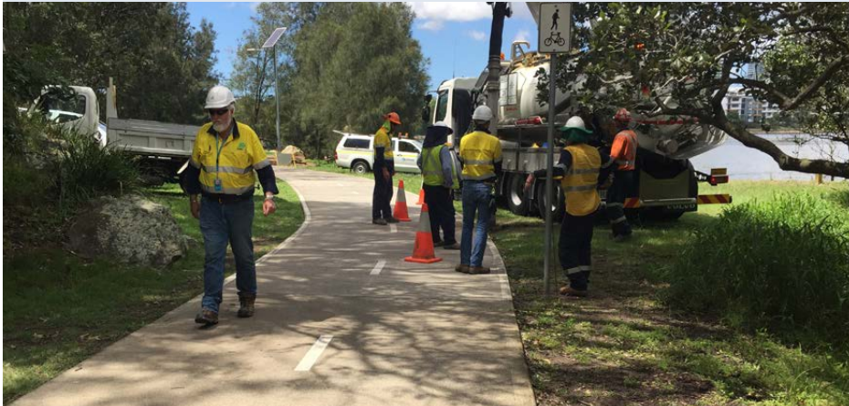
Marking the ground with temporary paint
