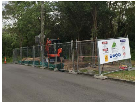
Maintenance and inspection activities on a section of a pipeline.
