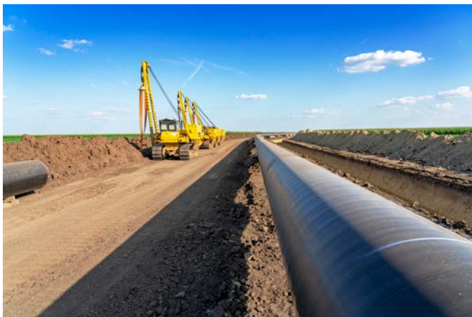
Pipeline maintenance works.
