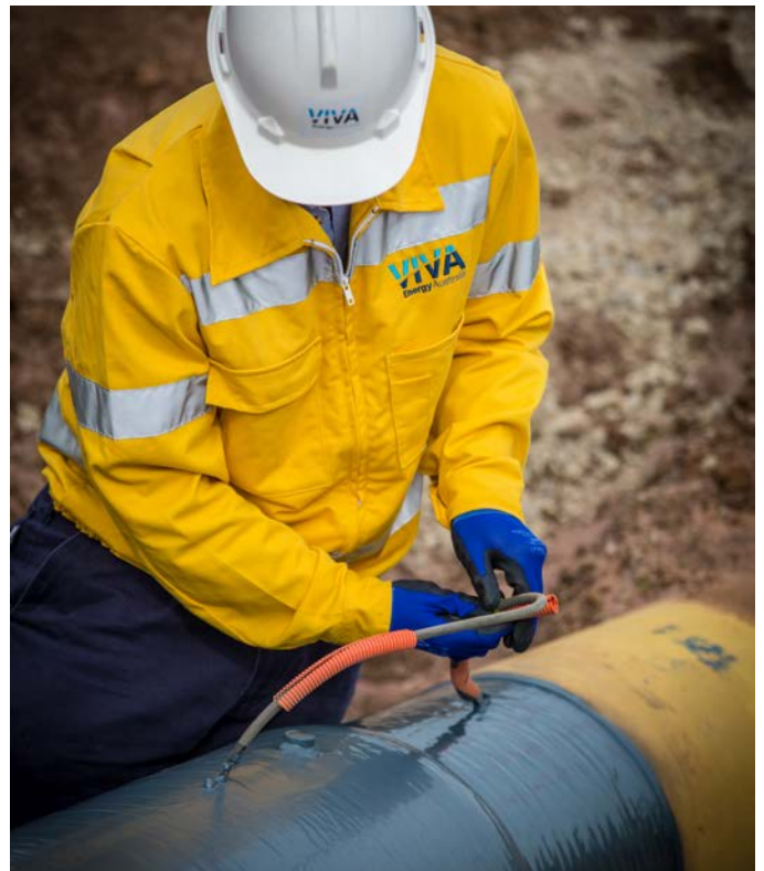
Maintenance works being carried out on a pipeline.
