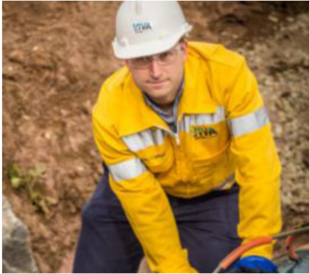
Maintenance and inspection activities being carried out on a section of a pipeline.
