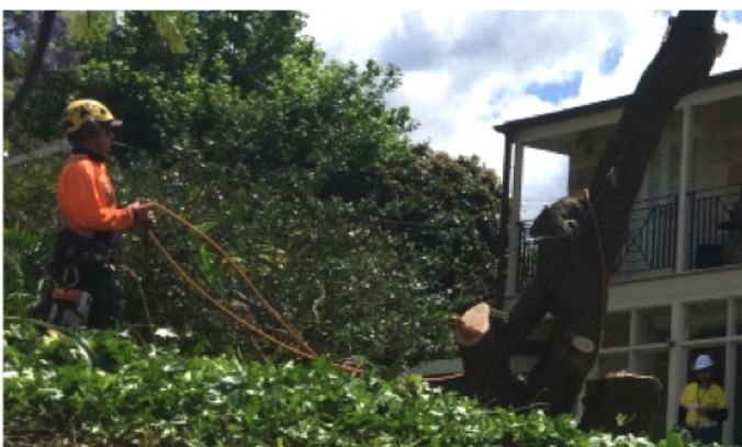
Tree removal works in progress ahead of pipeline maintenance works.
