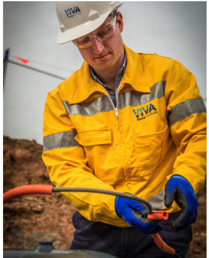
Maintenance works being carried out on a pipeline.
