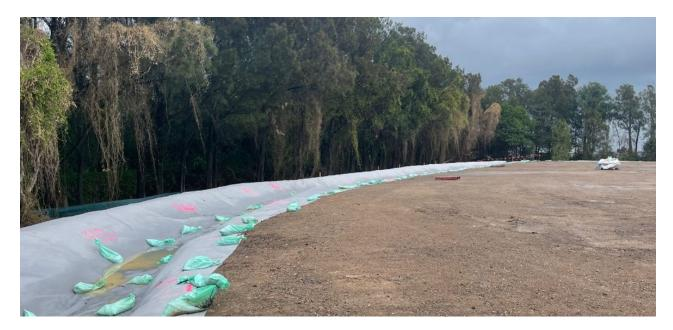
Photo 15 Stage 2 anchor trench (which will also allow future installation of services without disturbing the cap) with protection layer installed – southern perimeter. Unsealed soil is the prepared surface to be capped with the protection layer and the LDPE.
