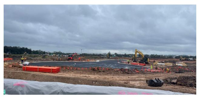
Photo 16 Northern boundary of containment cell in Lot 64 showing anchor trench and protection layer. Background is the cul de sac of the north-south road. Installation of service conduits
