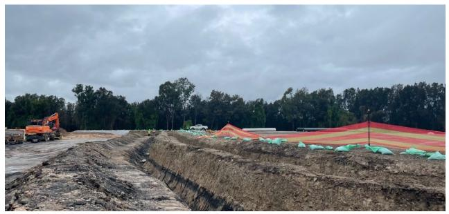
Photo 14 Stage 2 view of trench excavated for construction of northern retaining wall with anchor trench at foot of barrier mesh. Darker material at base of the retaining wall trench may be material buried within the containment cell
