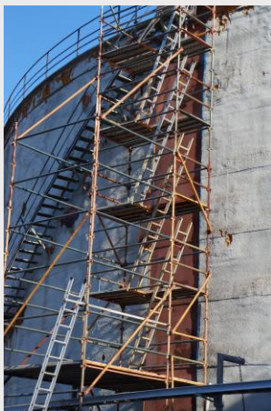
Cladding gradually being removed from a fuel oil tank.
