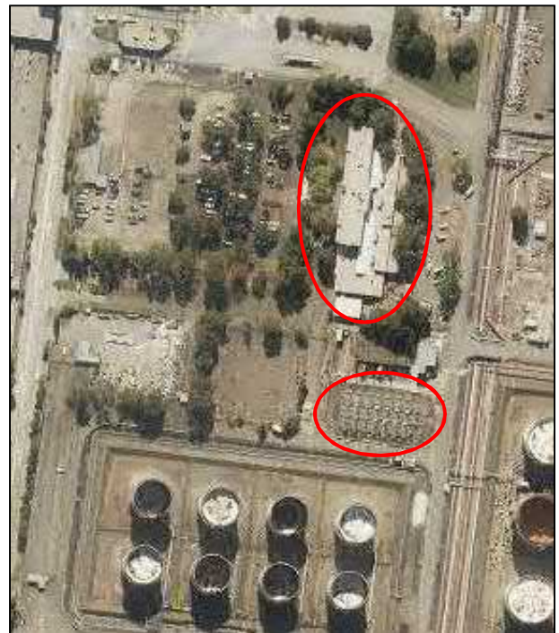
Figure 11: Current Aerial photo showing State Office Building and switchyard (Source: Sixviewer maps)
