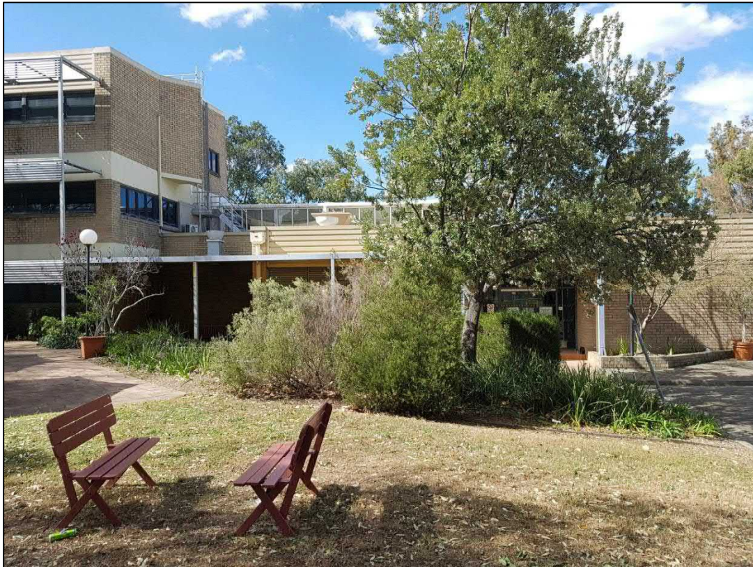
Figure 24: View of State Office Building looking east from carpark and entry off Durham Street showing single storey L shaped structure to south of building
