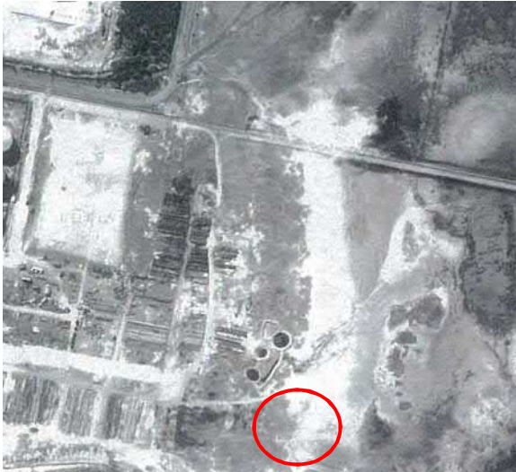
Figure 12: 1951 Part image of Aerial photo does not show the slops tanks (Source: Shell Australia)
