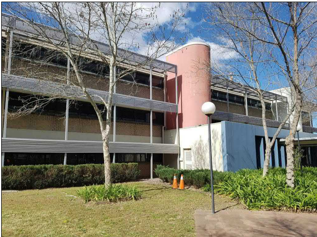
Figure 23: View of State Office Building entrance looking south east showing face brickwork, steel framed screen, stairwells and entrance
