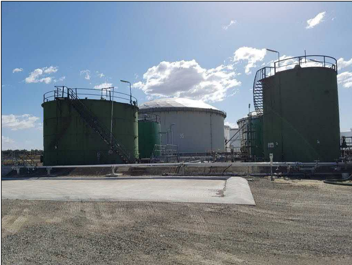
Figure 36: View of Tank T106 (slops tank) seen in the foreground to the left
