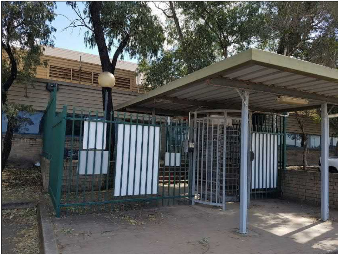
Figure 26: View of State Office Building looking west showing gated entrance, covered walkway and steps
