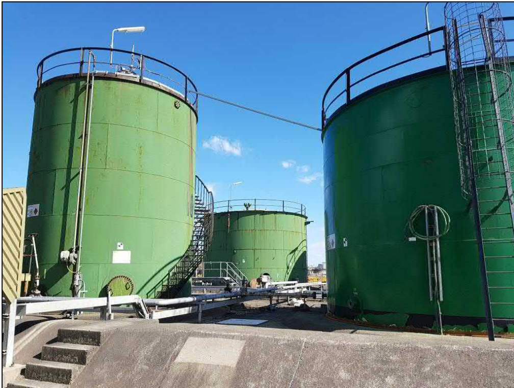
Figure 37: View of Tank T106 (slops tank) seen in the background
