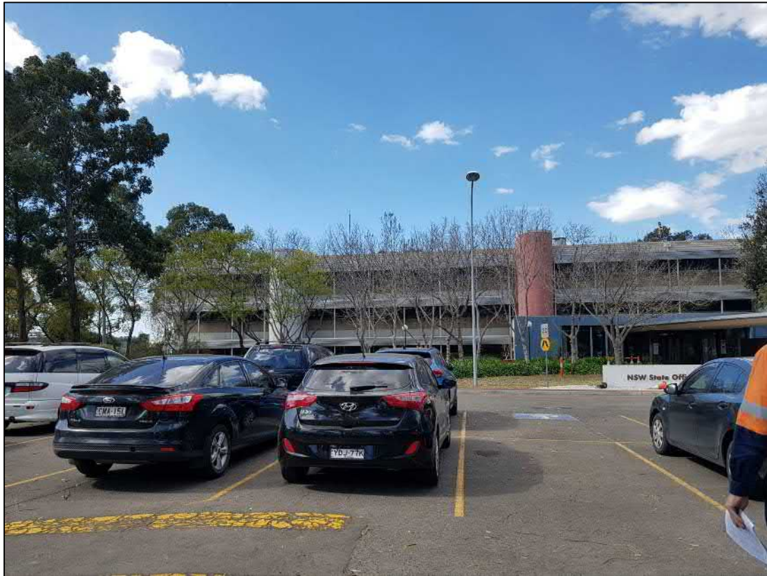
Figure 22: View of State Office Building looking east from carpark and entry off Durham Street
