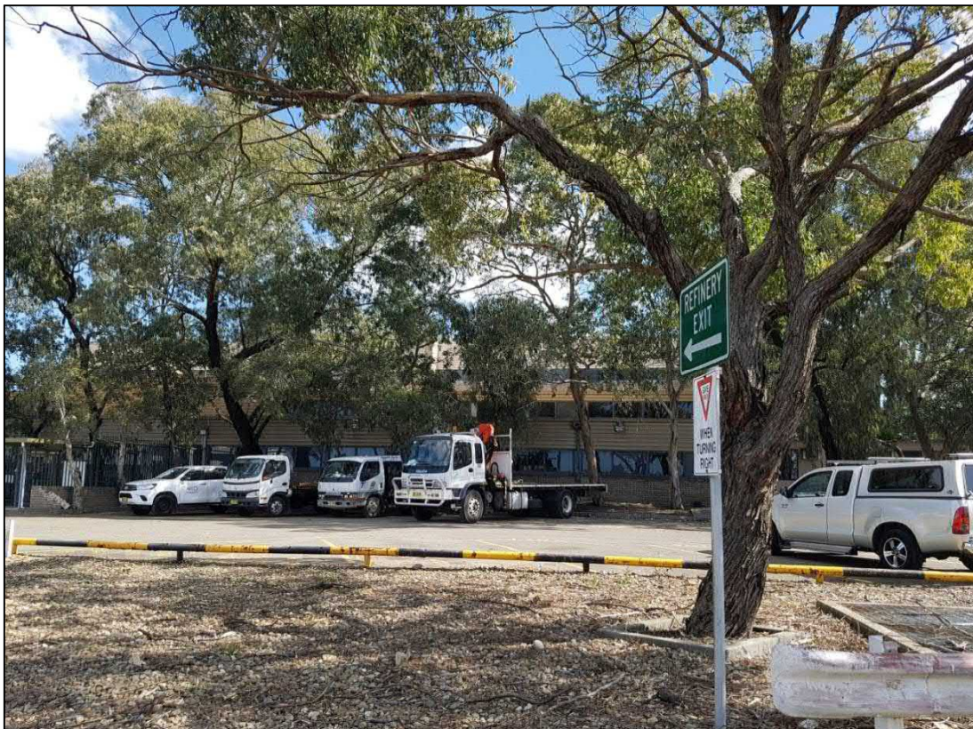
Figure 25: View of State Office Building looking west from carpark (rear of building) showing single storey building with skillion roof and clerestory windows
