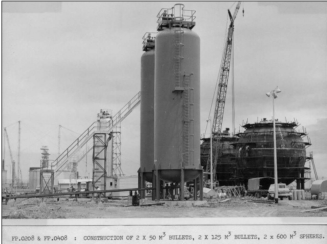
Figure 17: Construction of LPG spheres is seen in the background as early as 1962. These spheres appear to be those that are located east of V137 and V140 (Source: Shell Australia)
