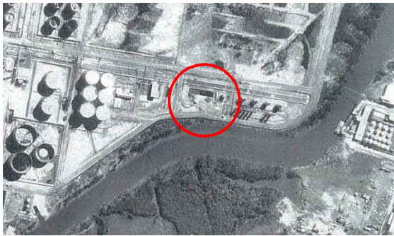
Figure 18: 1965 Part image of Aerial photo does not show any tanks in the location of V137 and V140 however, other cylindrical tanks are located to the east (Source: Shell Australia)
