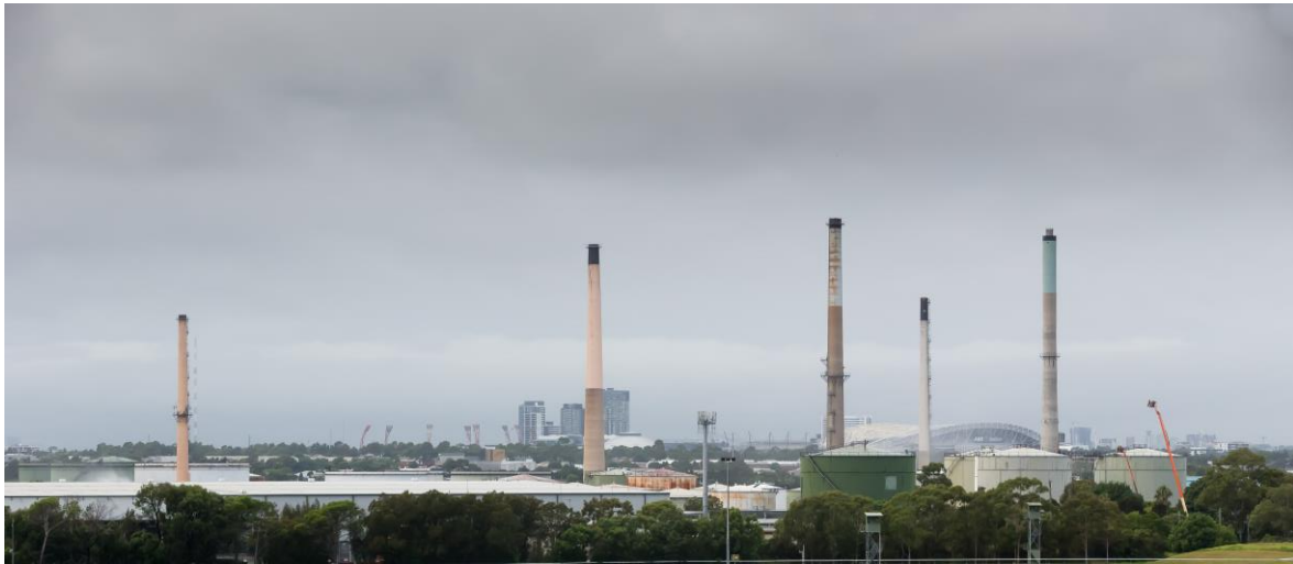
The five redundant chimney stacks before demolition, Sunday 21 February 2016
