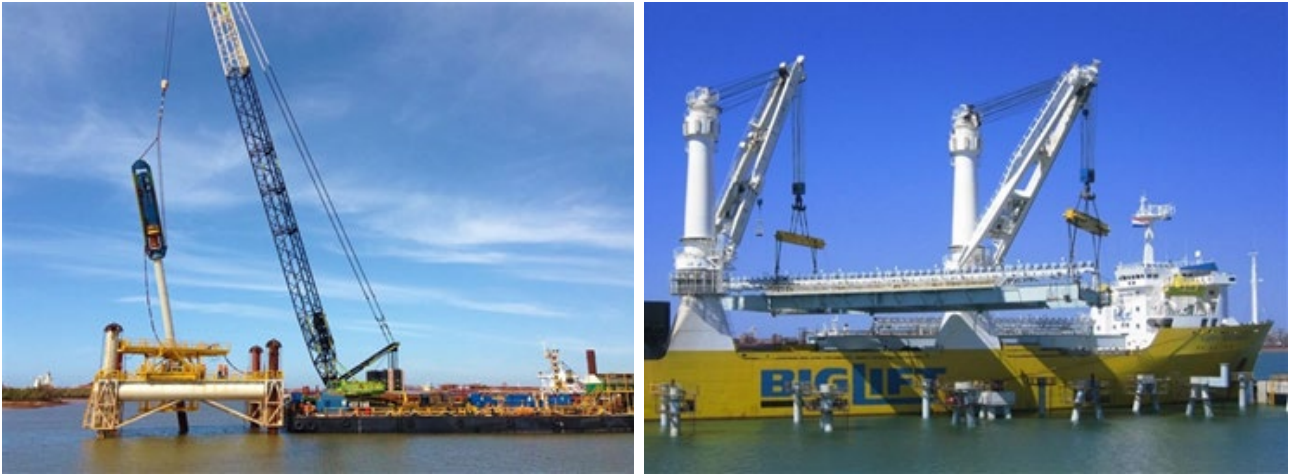
Figure 6 Example of pile driving (left) and installation of steel-fabricated module with heavy lift vessel (right)
