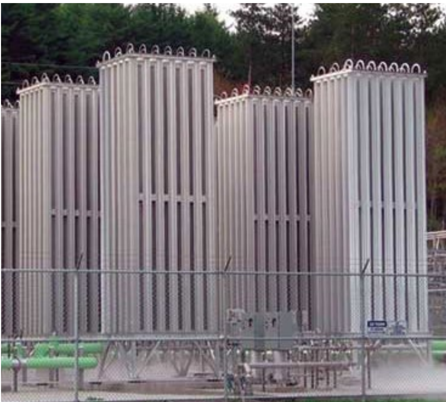
Figure 4-12 Ambient air vapourisers
