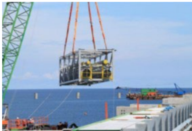
Figure 4-20 Installation of steel pipe rack with a crane barge
