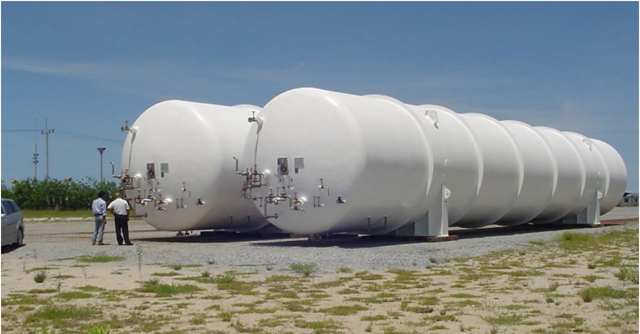
Figure 4-11 Horizontal liquid nitrogen storage vessels (source: Cryeng Group 2018)
