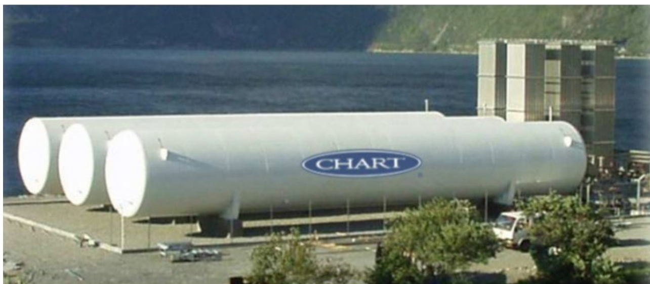
Figure 3-13 Example of VIV liquid nitrogen storage
