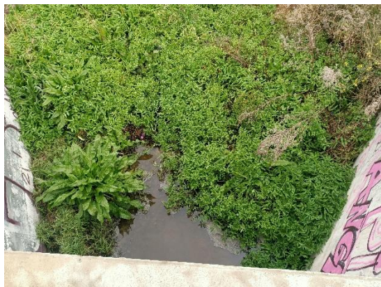
Close up of South Arm culvert showing extensive non-native macrophyte growth and stagnant water with surface film
